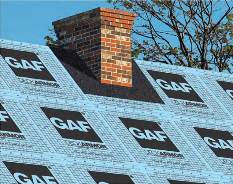
*Deck-Armor™ Premium Breathable Roof Deck Protection helps resist wrinkling and buckling for a more uniform look.*
