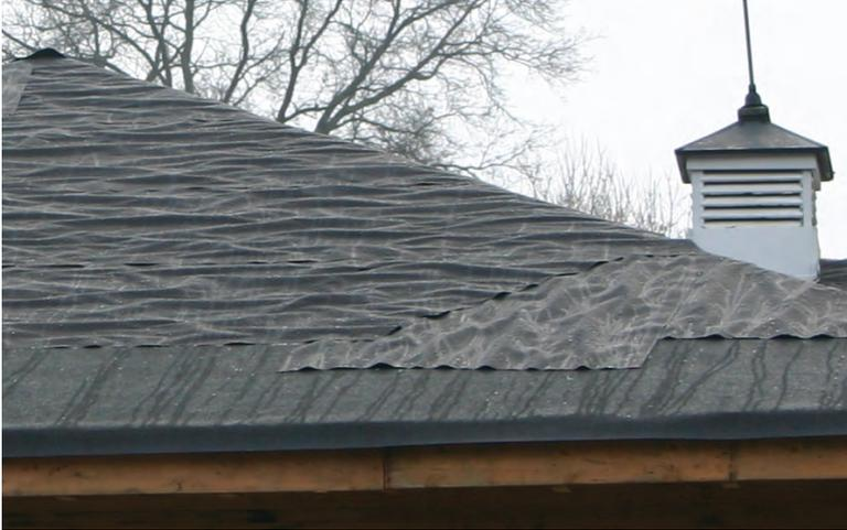
*Conventional organic felts can absorb moisture, causing buckling and wrinkling that can impact the look of your roof.*
