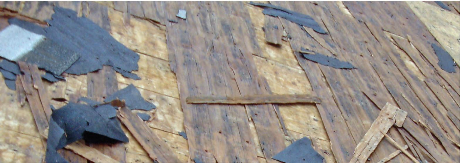
Today's modern homes are built weathertight — so common moisture (from cooking, bathing, cleaning, etc.) has less chance to escape. Over time, that can cause roof rot, mold, mildew, and costly structural decay.
